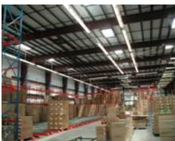
This 40,000 sq ft office/warehouse is equipped with a 20kW solar PV system. Part of the system is dedicated to the lighting and is integrated with occupancy and daylight sensors. Additional solar power is inverted and sent back to the grid. The low-cost DC ballasts, equipped with an internal occupancy sensor connection circuit, allow easy integration of the high efficiency controls.
